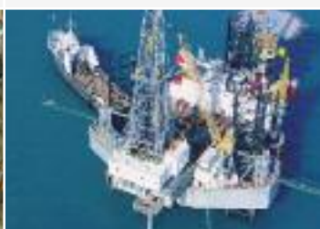
Raffinerie olio e gas
